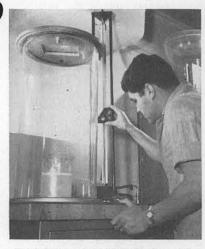
VACUUM CHAMBER IN AC-TION produces an atmosphere pressure euqivalent to 55,000 feet altitude as it sucks air out of a beaker of liquid plastic. The result is a clear plastic free from entrapped air. Lab assistant Benny Lucero, 1514-3, checks a reading on the vacuum gauge.
